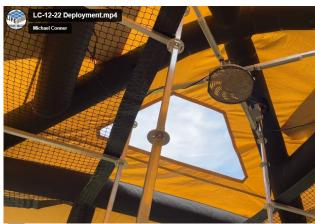
Robust frame construction and telescoping aluminum infrastructure. Skylights. Air circulation fan.
